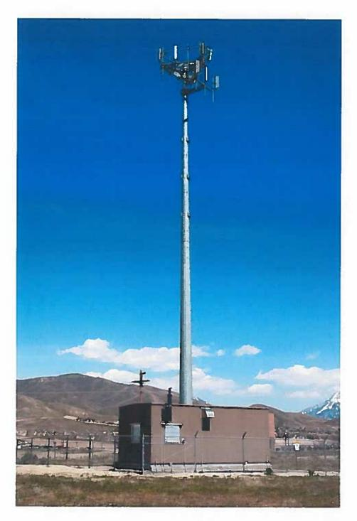
A single tubular mast up to 200 feet high with antennas mounted on the exterior. One of today's most widely deployed tower type.
