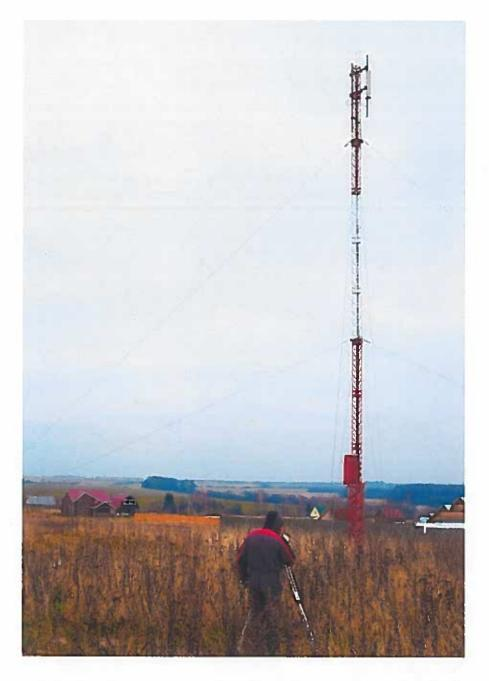
Similar to a monopole tower with a single mast, but stabilized with guy wires. Guy towers have been available to the industry for a long time and can be found in many configurations and situations. They range in size from 40 feet to over 2,000 feet for television and radio broadcast purposes.
