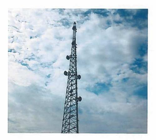
Often called a self-supporting tower; offers the most stability and flexibility of the cell tower types. Generally built with steel, and can have a square or triangular shape. Many of the original communications towers were self supporters and can be found as tall as 500 feet.
