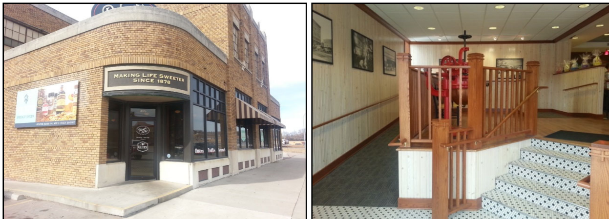
Fig. 4-8. Example of structure before (left) and after (right) first floor elevation.
