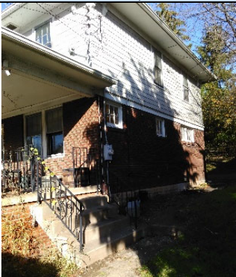
Front Side View, Southwest
