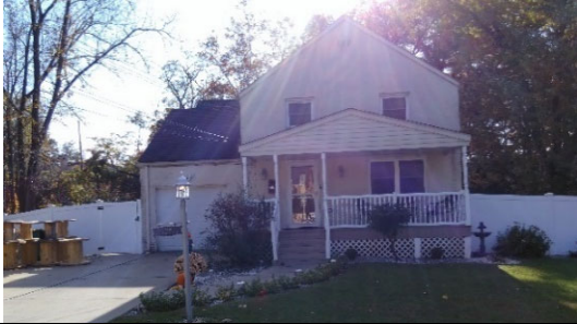
Front View, Northwest
