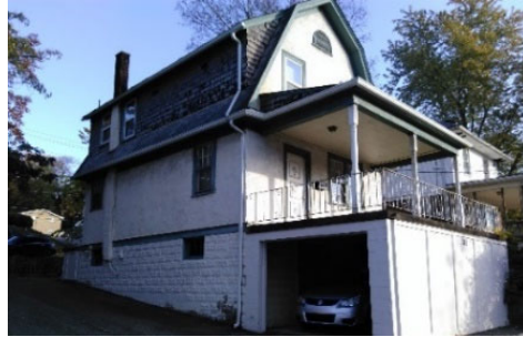
Side View, Southwest
