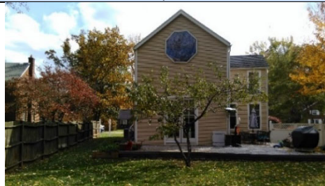
Rear View, Northwest
