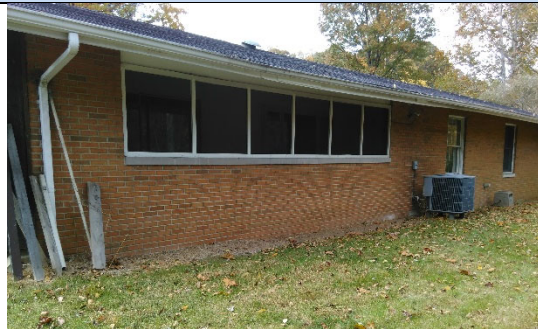
Rear View, Northwest
