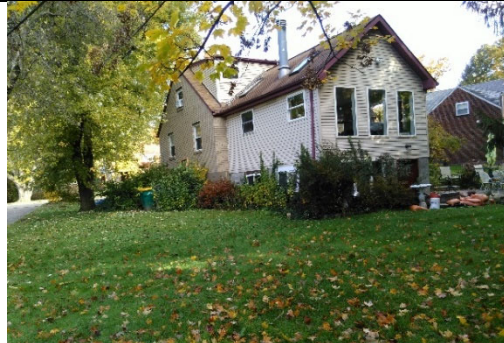
Rear View, Southwest
