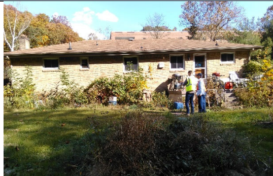
Rear View, West
