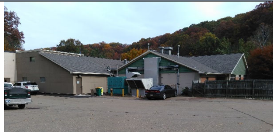
Rear View, West
