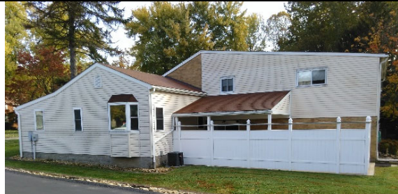
Side View, Southwest
