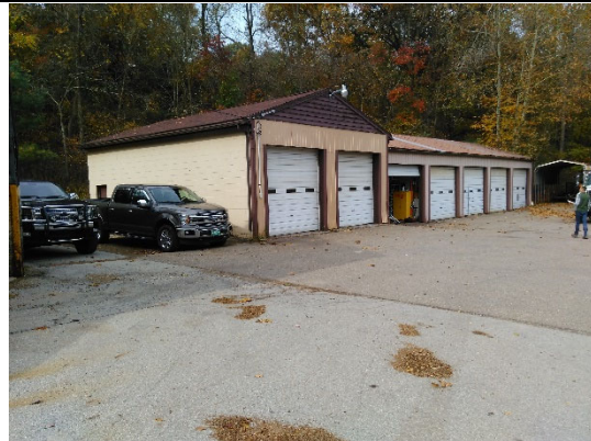
Front Side View, Southeast
