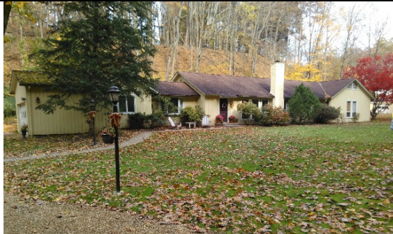
Front View, Southeast
