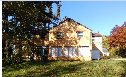
Rear View, East
