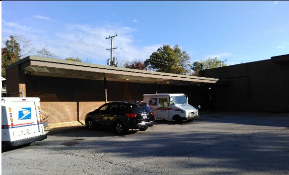
Side View, Southwest
