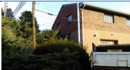
Side View, Southeast
