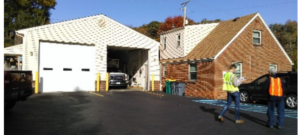
Rear View, Southeast
