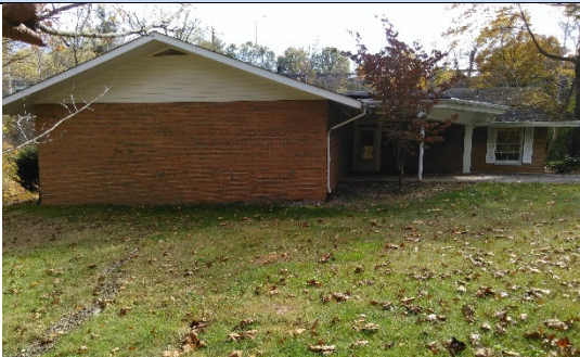
Side View, North
