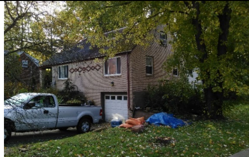
Front Side View, Northwest
