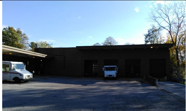
Side View, West
