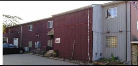
Rear View, Northwest
