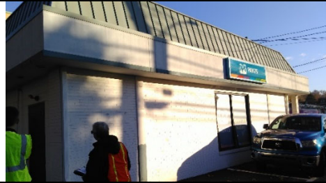
Side View, South
