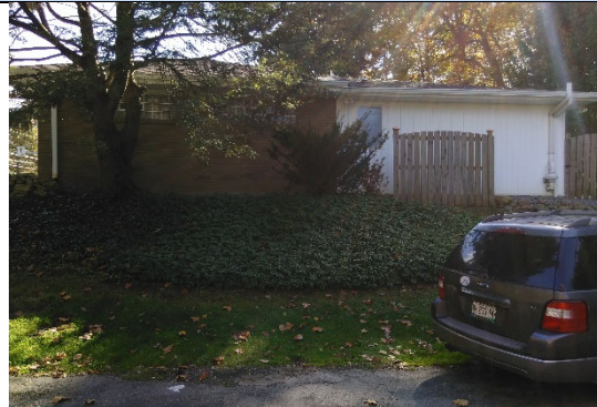
Rear View, West
