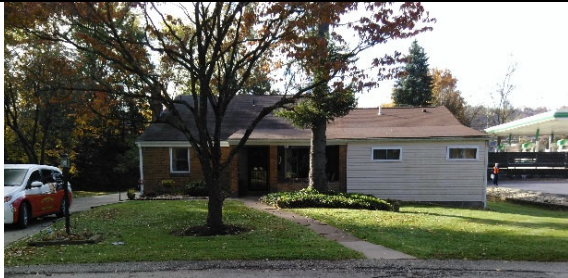
Front View, North
