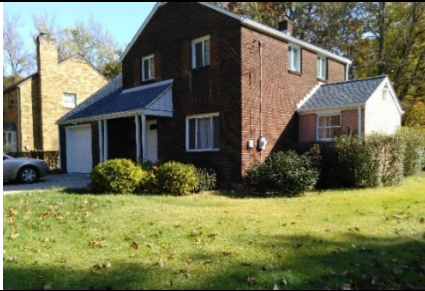
Front View, Southwest
