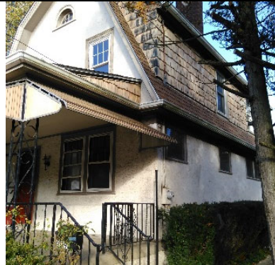
Front Side View, Southeast
