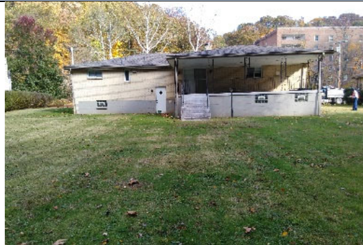
Rear View, West
