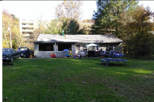
Rear View, West
