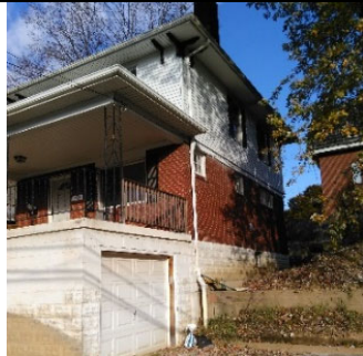
Front Side View, Southeast
