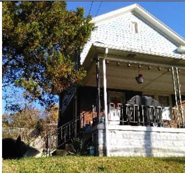
Front Side View, Southwest
