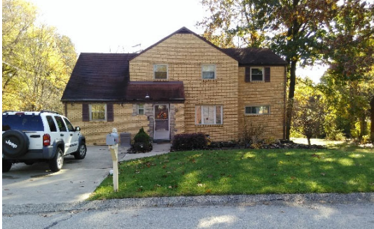
Front View, West
