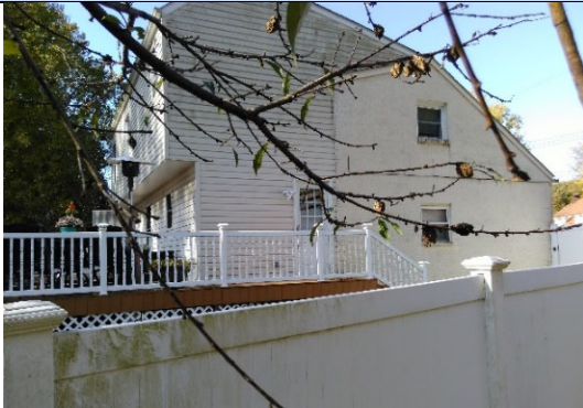
Rear Side View, East
