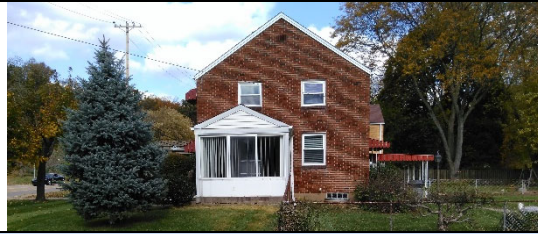
Side View, West
