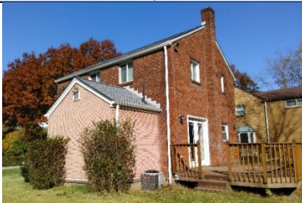
Side View, Southeast
