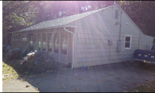
Front Side View, Northeast
