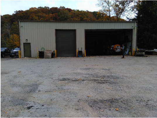
Front View, West
