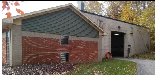
Side View, North
