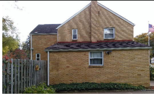
Side View, North
