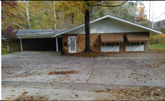
Front View, West
