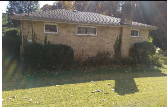
Side View, North
