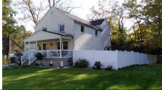
Side View, West
