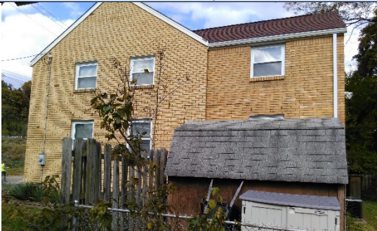
Side View, South
