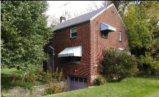
Front View, Southwest
