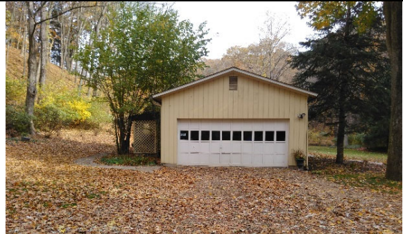
Side View, Southwest
