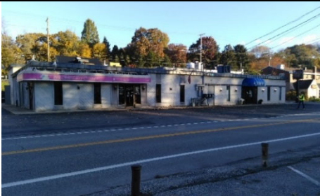
Front View, North
