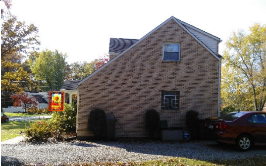
Side View, North
