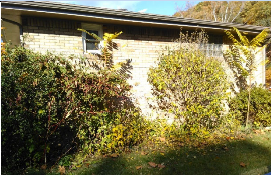
Side View, South
