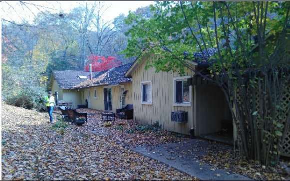
Rear View, Northwest
