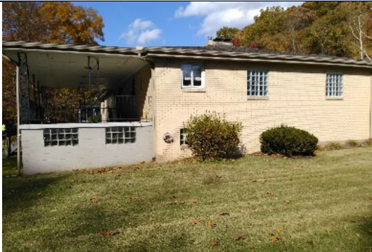
Side View, South
