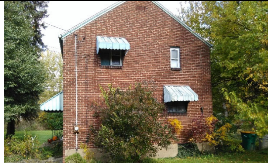
Side View, South
