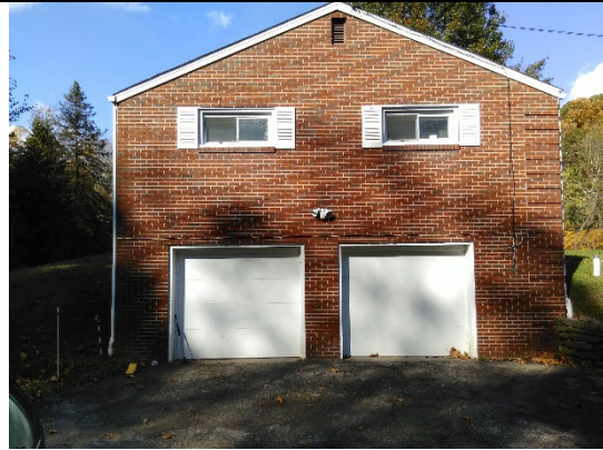
Side View, South
