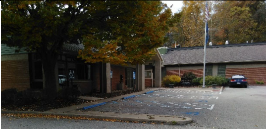
Front View, Northeast
