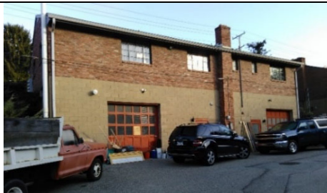
Rear View, Southwest
