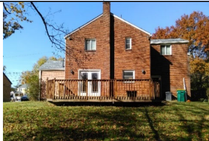
Rear View, East
