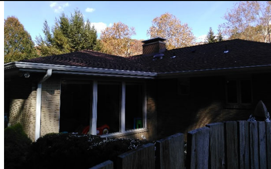
Side View, Southeast
