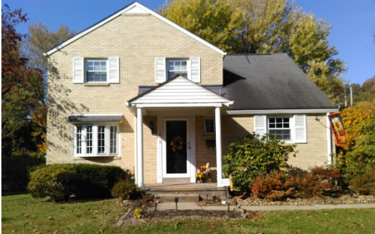
Front View, Southeast
