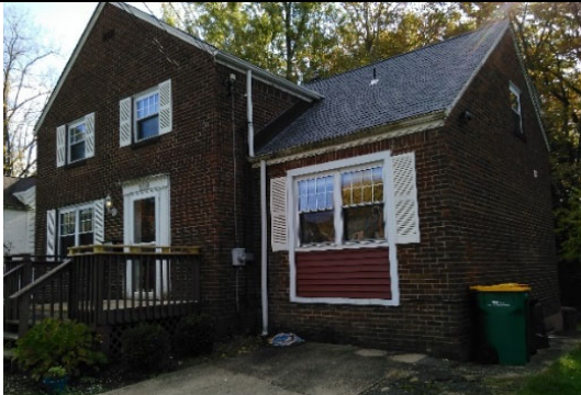
Front View, Northwest
