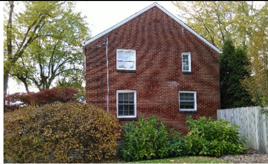
Side View, Southeast
