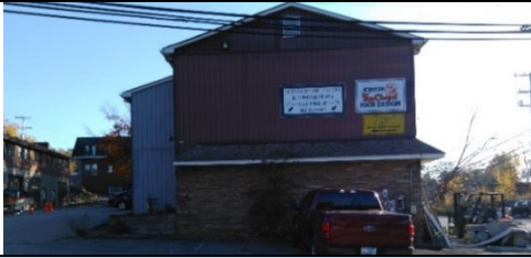
Side View, West
