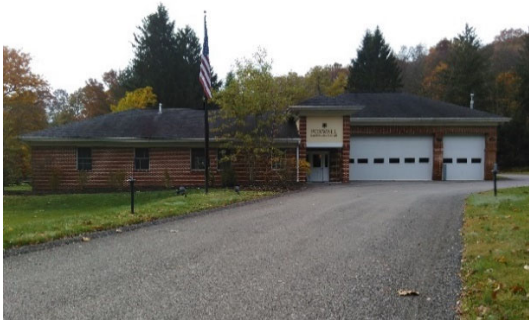
Front View, North
