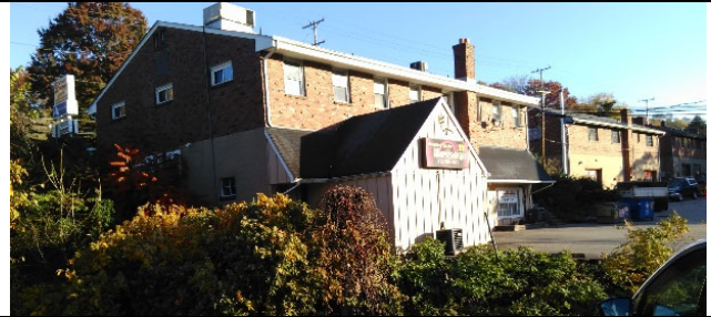
Side View, Southwest
