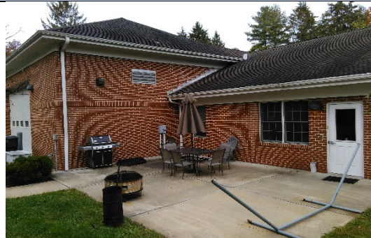
Rear Side View, Southeast
