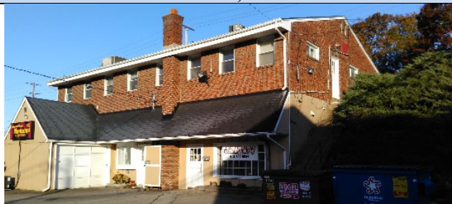
Side View, Southeast
