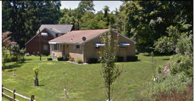
Side View, North
