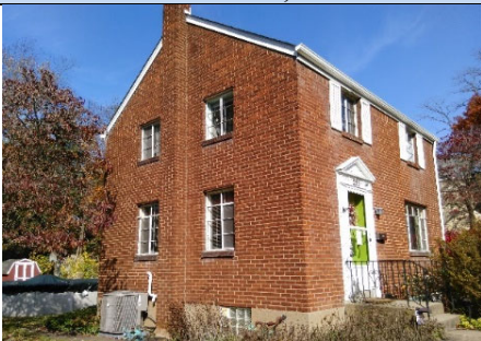
Side View, Southeast
