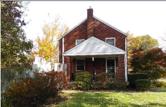
Side View, West
