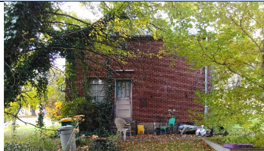
Rear View, East
