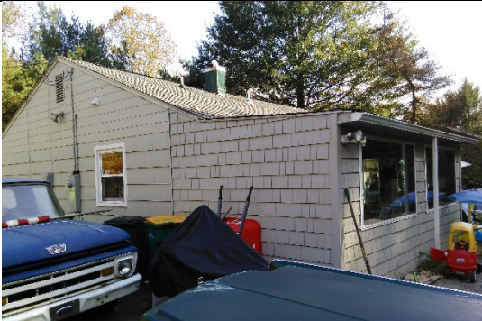
Side View, Southwest
