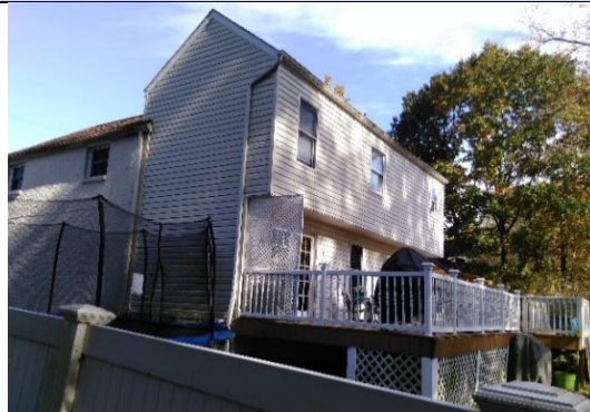
Rear View, South
