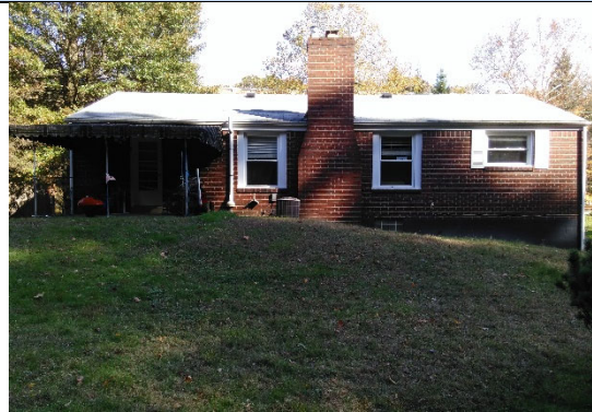
Rear View, West
