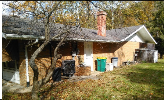
Side View, Southwest
