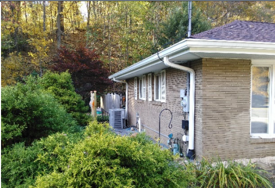
Side View, Southeast
