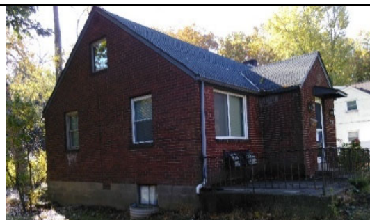
Side View, North
