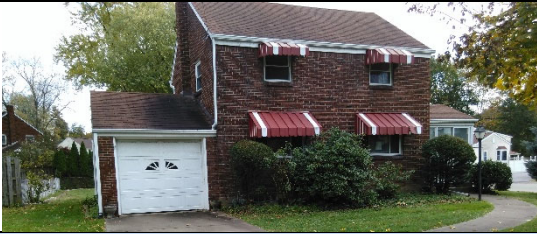
Front View, Northwest
