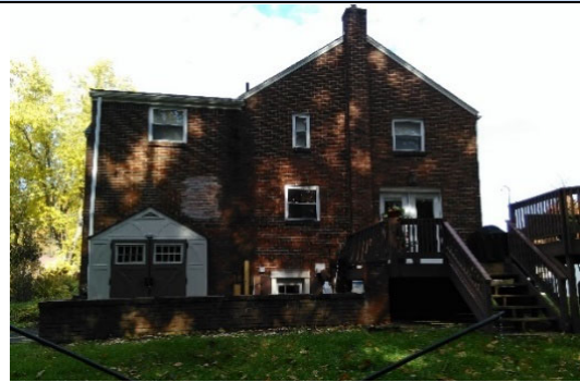
Rear View, South
