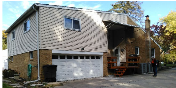
Rear Side View, Southeast
