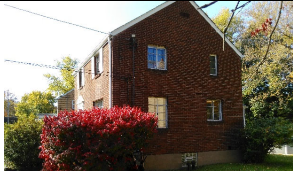
Side View, North
