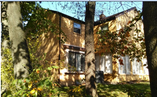
Side View, Southeast
