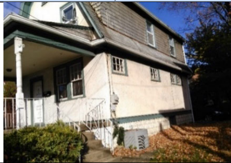
Side View, Southeast
