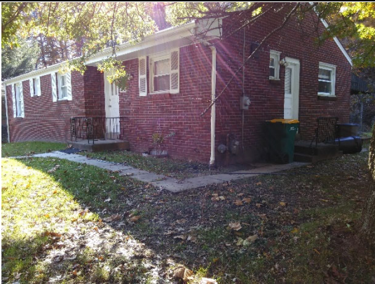
Front View, Northeast
