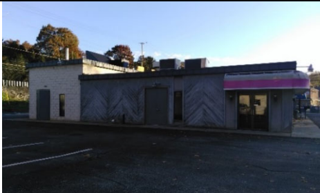
Side View, West
