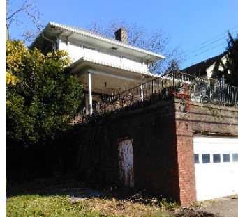
Front Side View, Southwest
