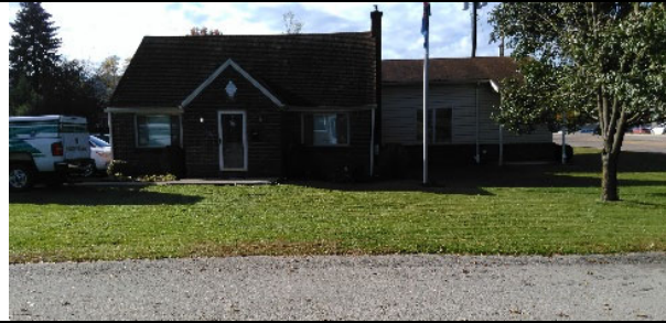
Front View, North
