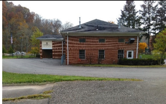
Side View, West
