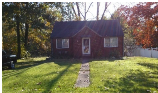
Front View, Northwest
