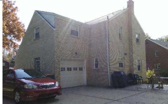
Rear View, Northwest
