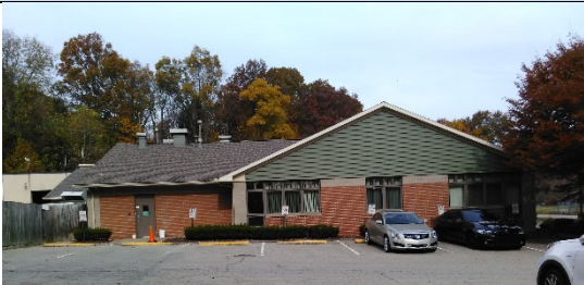
Side View, South
