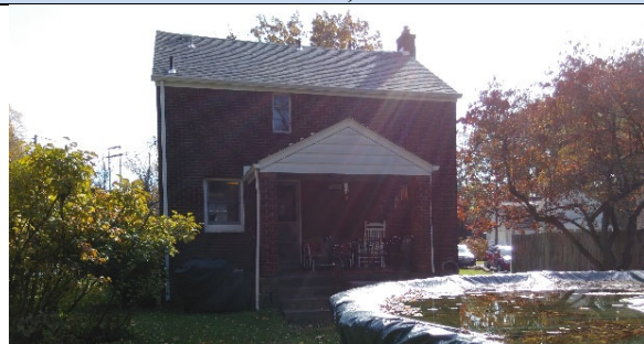
Rear View, West
