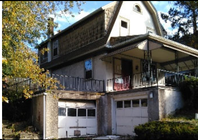
Front Side View, Southwest
