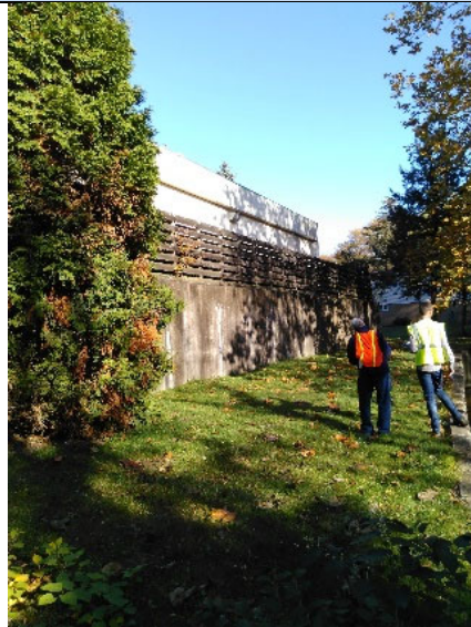
Rear View, Southeast
