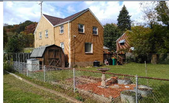
Rear View, Southeast
