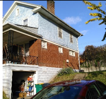
Front Side View, Southeast
