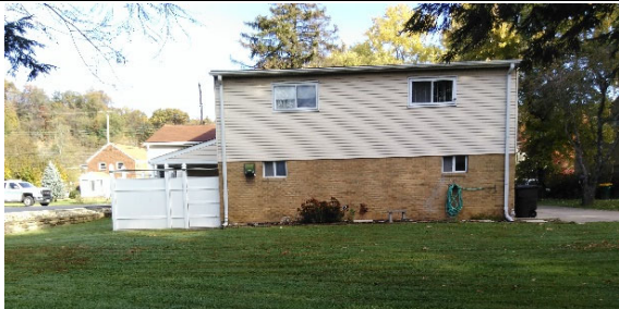
Rear Side View, South
