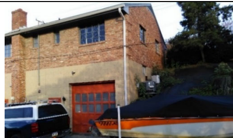
Side View, South
