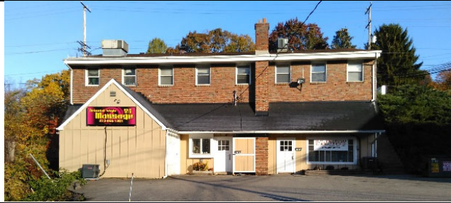
Rear View, South
