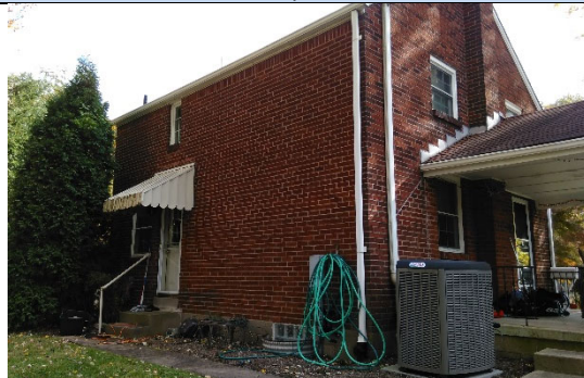
Rear View, Northwest
