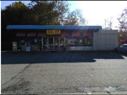
Front View, West
