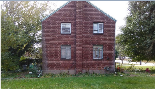
Side View, North
