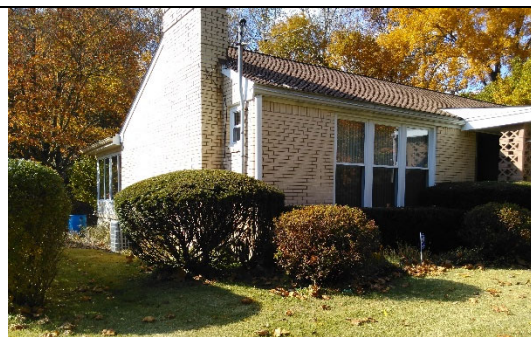
Front Side View, Southeast
