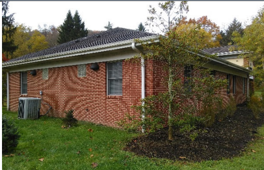
Rear View, East
