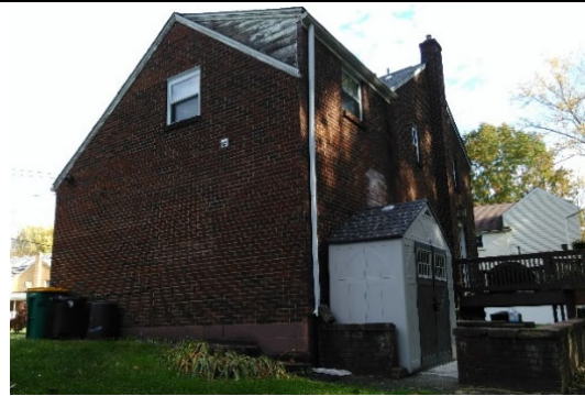
Side View, Southwest
