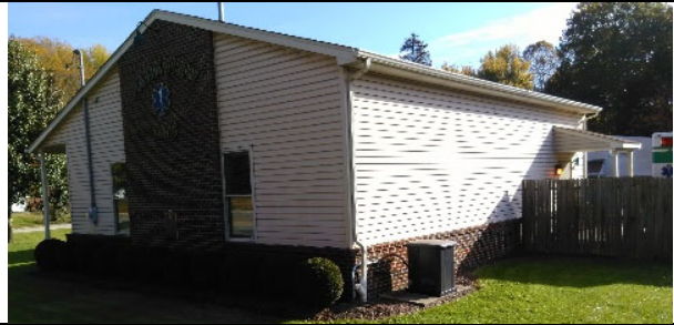
Front Side View, Southwest
