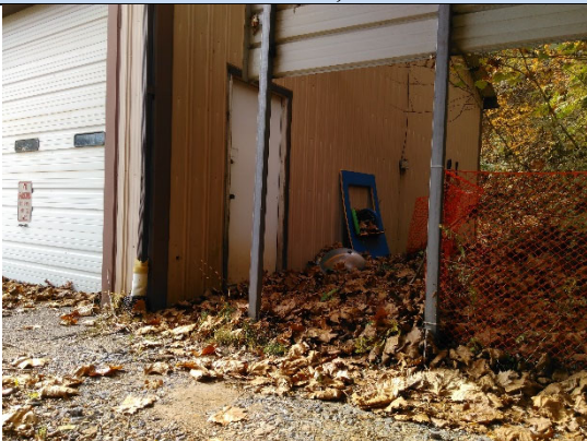
Front Side View, Northeast
