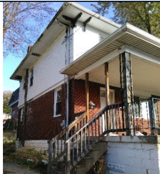
Front Side View, Southwest
