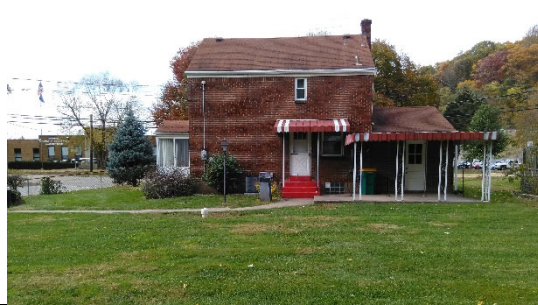
Rear View, East
